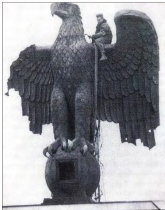
The Massive Tempelhof Airport Eagle. Originally the main building had an eagle sitting atop the globe - this remained until the 1960s when it was scrapped. Only its head remains. It was designed by Albert Speer in 1936. From FB June 2025: History & Military II... Photographer unknown
